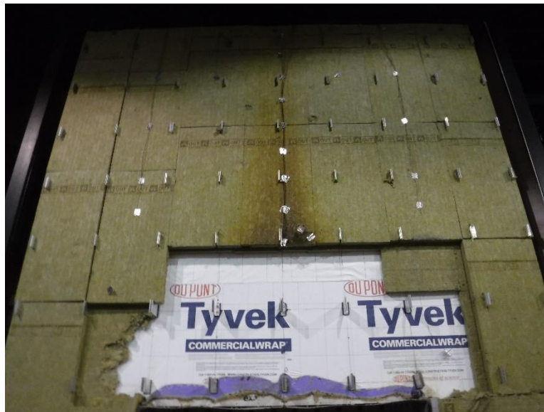
Photo No. 23 Mineral Wool Removed
