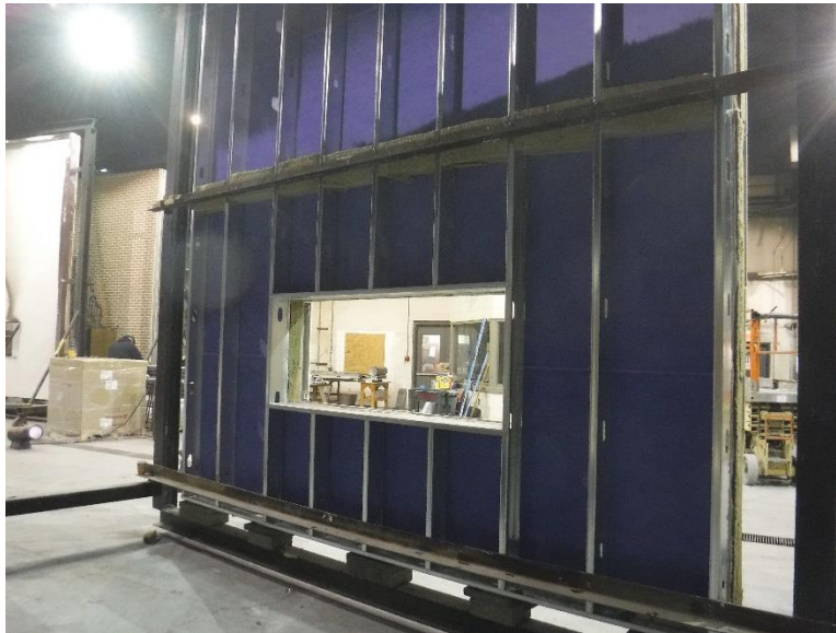
Photo No. 11 Safing Installed
