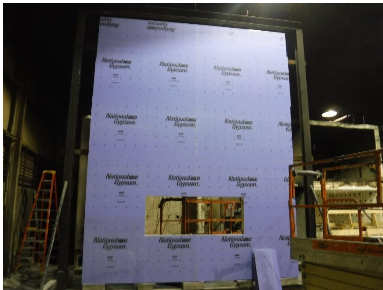
Photo No. 2 Exterior Sheathing Installed
